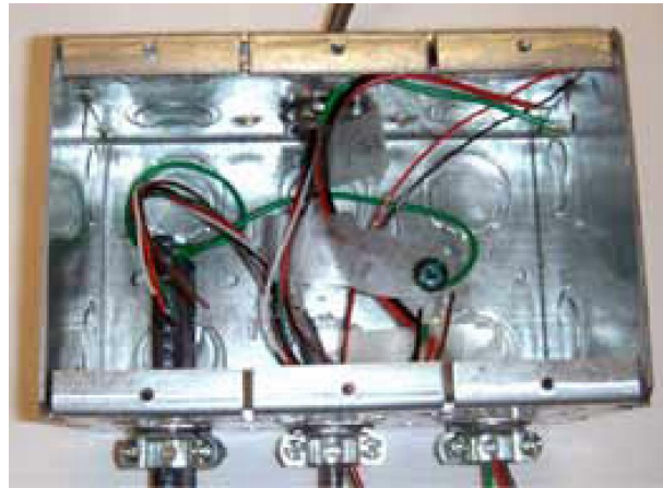
Tripe gang electrical box rough wiring and plumbing
